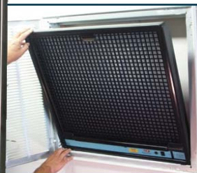
FG EAC Model shown installed into a 1" R/A Filter Grille
